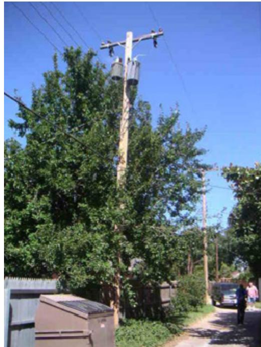
This pole, maintained by LP&L, just two streets away from Edwards' home, is a significant source of harmful interference coming from this general area, according to Gruber. This source also has a signature that clearly matched a component of the interference from Edwards' home. The actual source of the noise is in the area of the insulator on the left side (field phase) of the cross arm. An adjacent property owner reports she is unable to listen to radio broadcasts as a result of interference.
