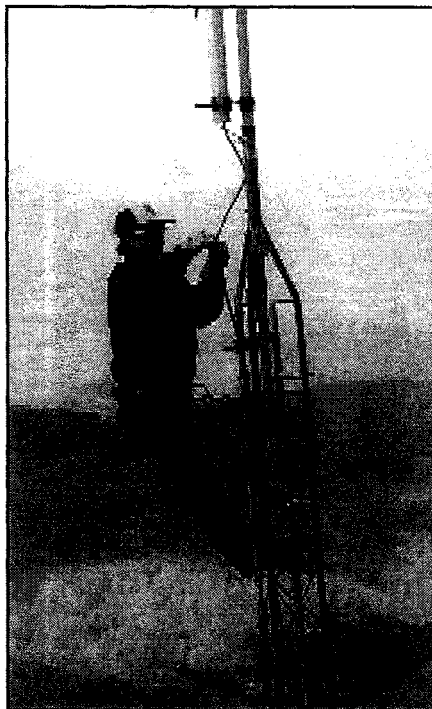
Figure 5.2—This repeater antenna is not mounted on a building and is located more than 10 meters above ground, so the operator of the repeater is not required to do a routine station evaluation.
