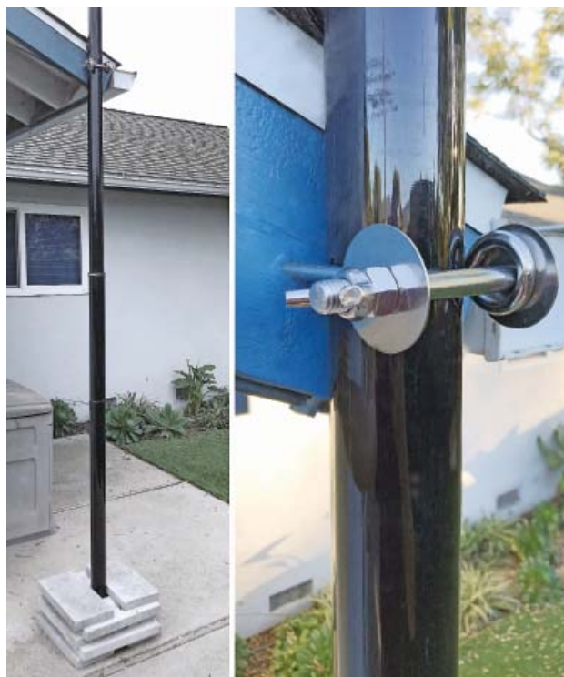
Figure 4 — What the mast looks like once it's mounted to the eaves. Note the stack of heavy patio bricks holding the mast in place.
