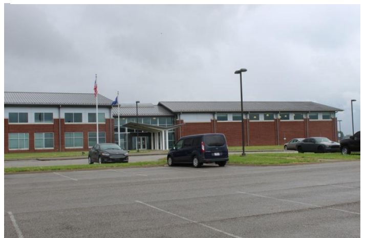
Figure 4 National Guard Armory - Daviess Co Dist 2 office
